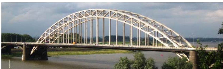
The 1936 Waal Bridge, famed for its WWII role in Operation Market Garden.
